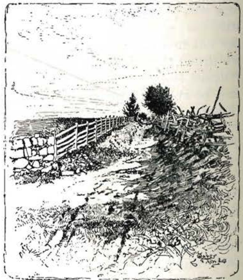
THE SUNKEN ROAD, LOOKING EAST FROM ROULETTE'S LANE. FROM A PHOTOGRAPH TAKEN IN 1885.
